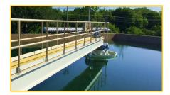
Clarified water is separated from fine sediments in the water by filters that remove any remaining suspended particles in the water. Then, treated water is disinfected and stored in water storage tanks that allow time for the chemicals to mix throughout the water.
